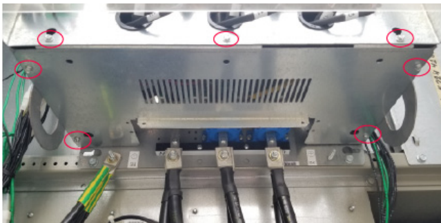
Figure 5. Removing drive chassis sheet
