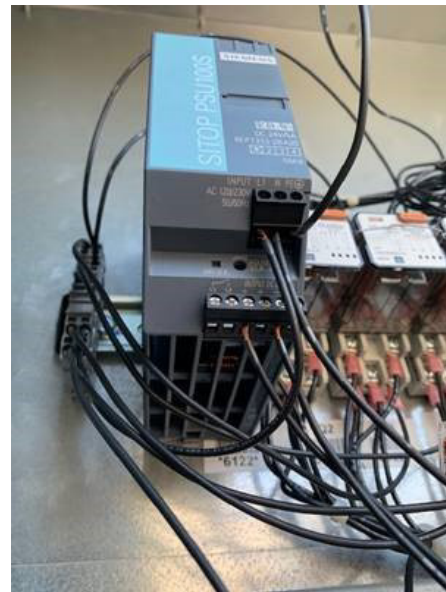
Figure 7. Installing additional terminal block
