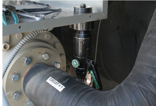
Figure 60. Create compressor conduit connection point
