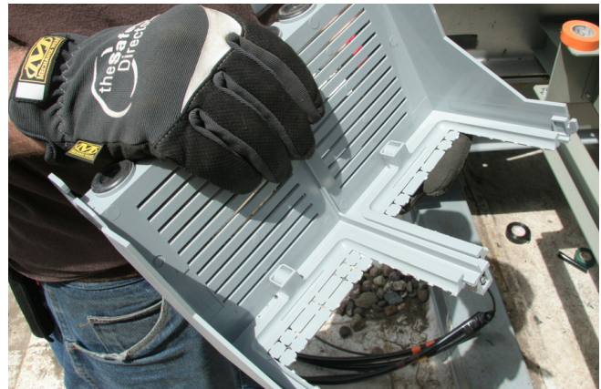
Figure 58. Touch safe cover installed
