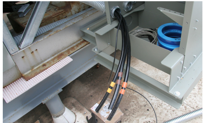
Figure 51. Install conduit at AFD enclosure
