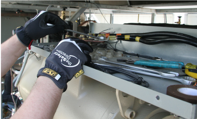
Figure 63. Connect wires to motor terminals
