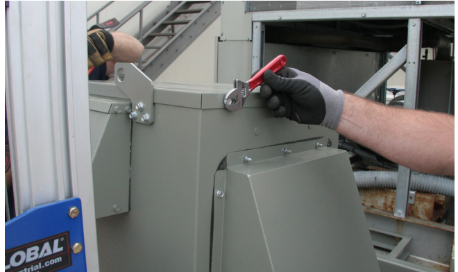
Figure 27. Remove top cover of enclosure
