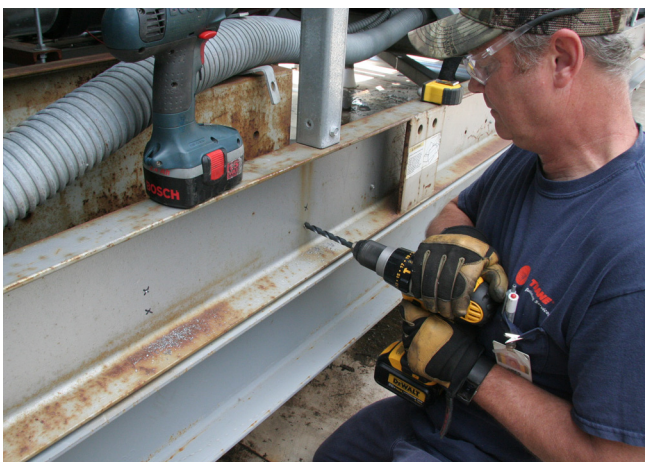
Figure 20. Drill 5/8-inch holes in base
