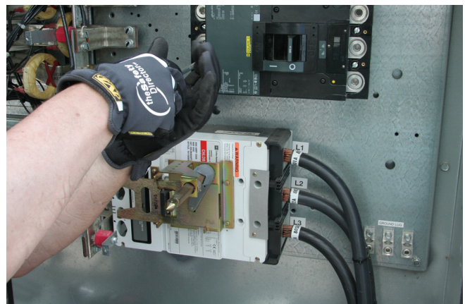
Figure 43. Install circuit breaker
