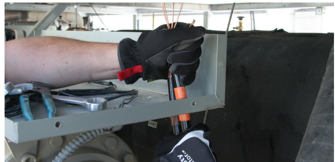
Figure 62. Install conduit at compressor
