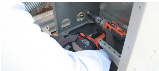
Figure 50. Create AFD conduit connection
