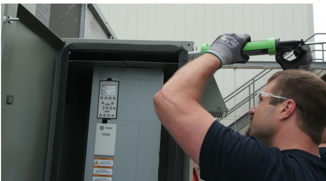
Figure 39. Apply sealant
