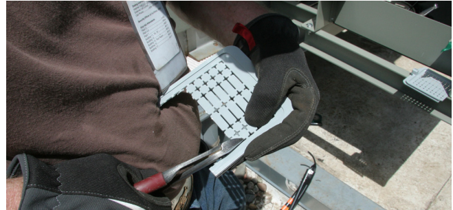
Figure 56. Touch safe cover sizing
