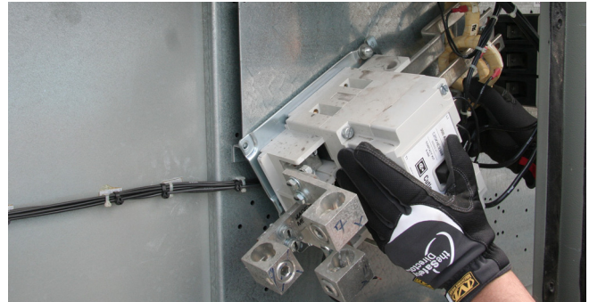
Figure 42. Contactor left in place
