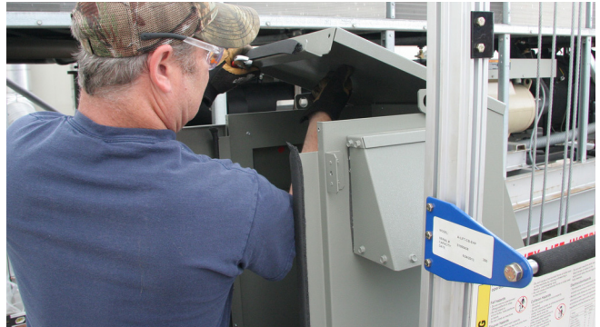
Figure 27. Remove top cover of enclosure
