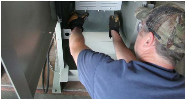
Figure 25. Remove bottom airflow duct
