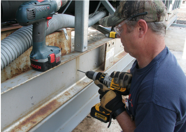
Figure 20. Drill 5/8-inch holes in base
