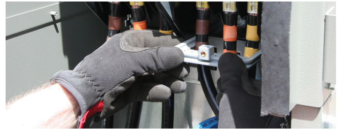
Figure 56. Touch safe cover sizing
