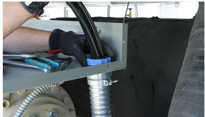
Figure 62. Install conduit at compressor
