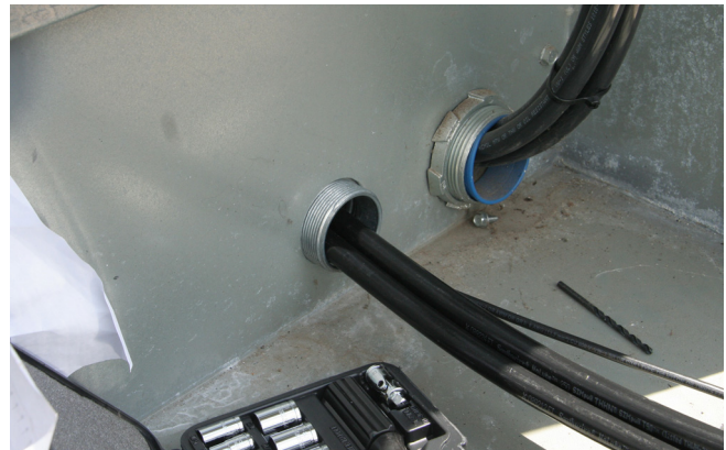
Figure 48. Route power wire to AFD
