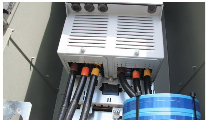
Figure 58. Touch safe cover installed
