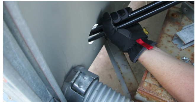
Figure 48. Route power wire to AFD
