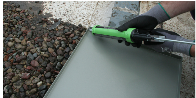
Figure 36. Apply caulk
