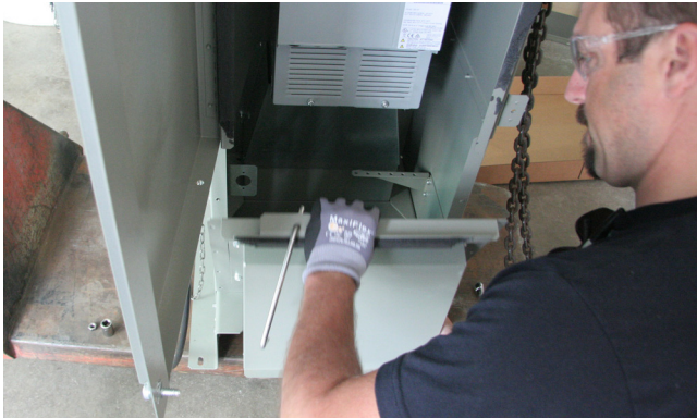
Figure 24. Remove access panel
