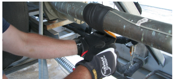
Figure 72. Sensor covered with insulating tape
