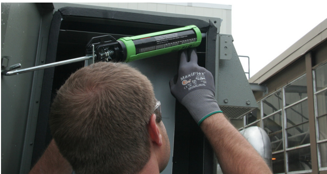
Figure 38. Apply sealant
