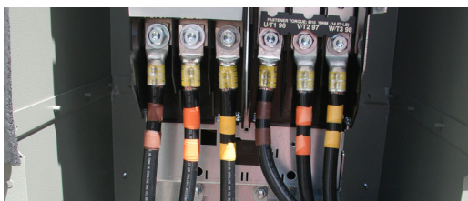
Figure 54. Install output wire at AFD
