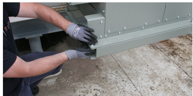
Figure 22. Attach enclosure to mount
