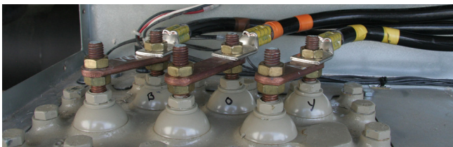
Figure 64. Install shorting bars for wye-delta starters
