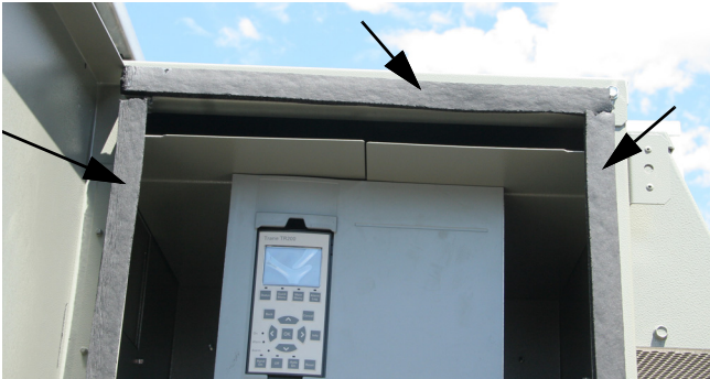
Figure 37. Gasket installed
