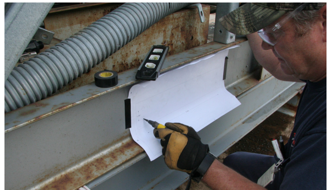
Figure 18. Mark drilling locations with template
