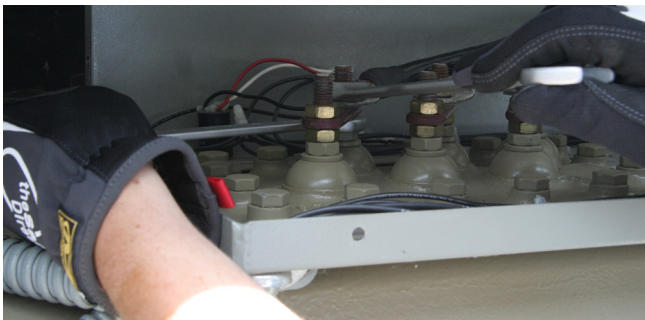
Figure 59. Remove compressor wiring
