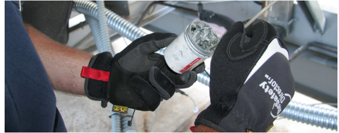
Figure 70. Use thermal paste on sensor
