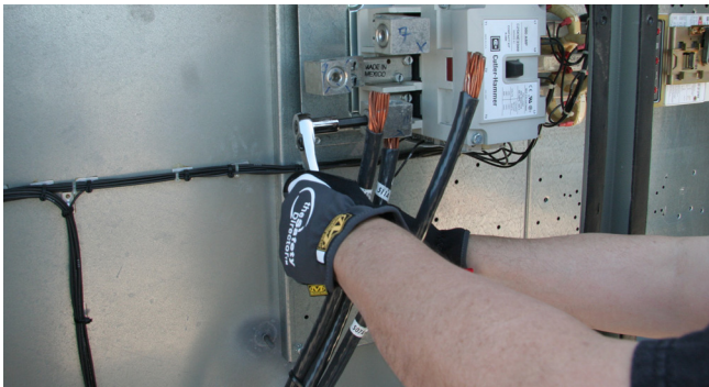
Figure 40. Remove compressor wire
