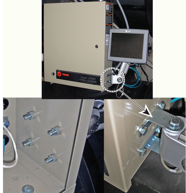
Figure 4. Bolting display arm to the panel
