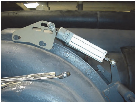
Figure 11. Installed stepper IGV actuator
