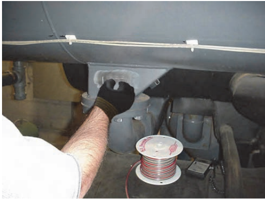
Figure 9. Sensor mounting with Armaflex insulation
