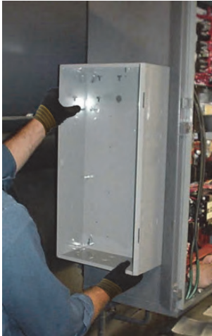
Figure 45. Mounting starter sub-box
