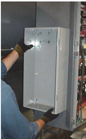
Figure 50. Mounting starter sub-box
