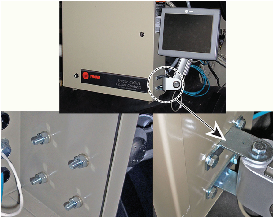
Figure 7. Bolting display arm to the panel
