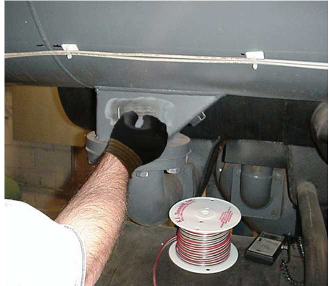
Figure 12. Sensor mounting with Armaflex insulation
