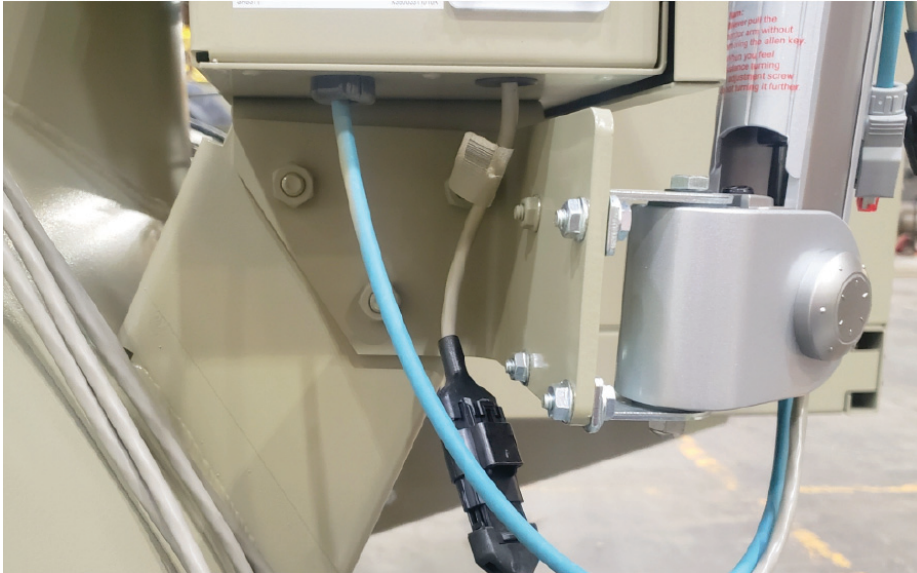
Figure 7. Bolting display arm to the panel
