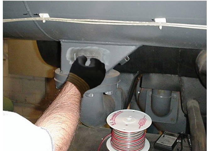
Figure 13. Sensor mounting with Armaflex insulation
