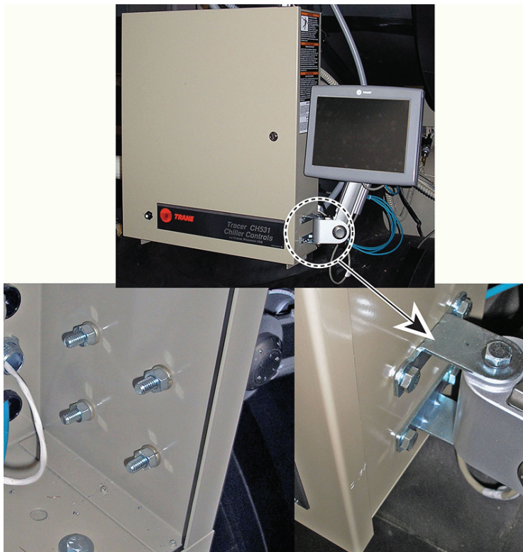
Figure 8. Bolting display arm to the panel
