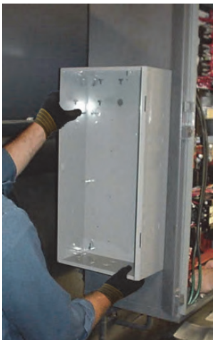
Figure 49. Mounting starter sub-box
