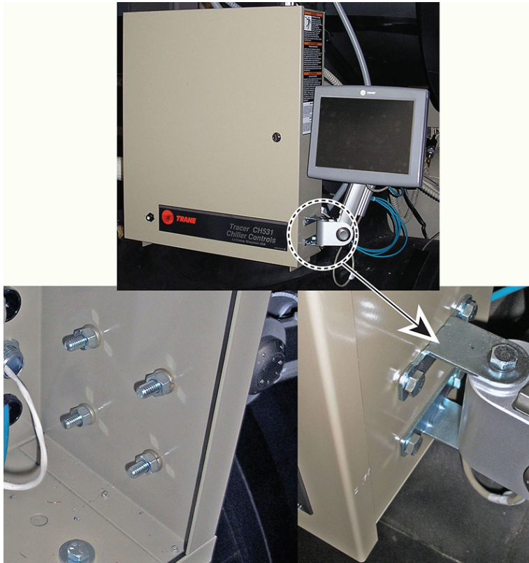
Figure 7. Bolting display arm to the panel
