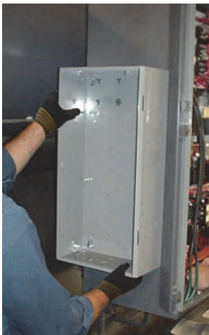
Figure 48. Mounting starter sub-box
