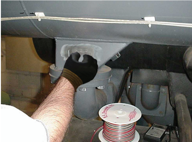
Figure 12. Sensor mounting with Armaflex insulation
