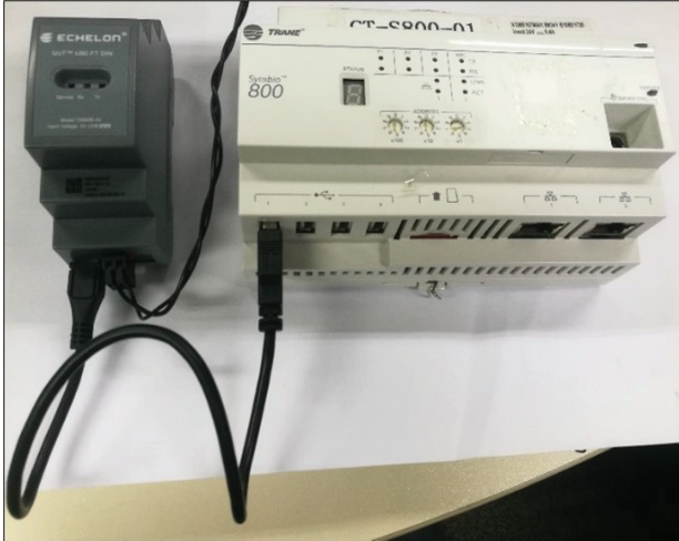
Figure 19. LON wiring, ref. 50712732
