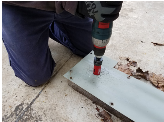
Figure 15. Wire routing hole creation
