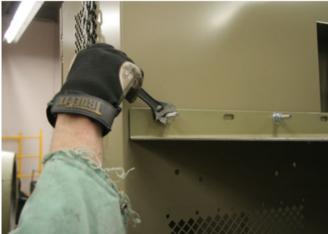
Figure 21. Attaching the Z-bracket at the top of the panel
