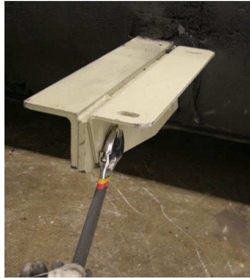
Figure 15. Removing bottom panel bracket from starter panel brackets
