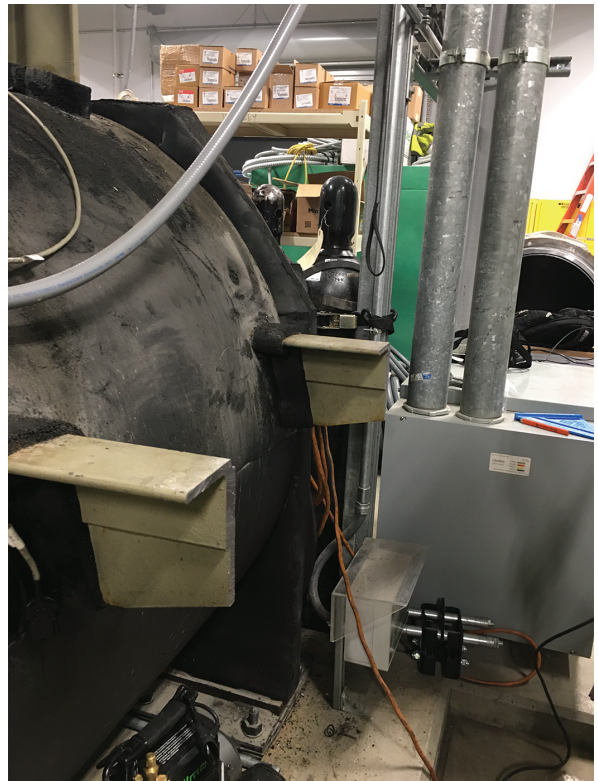
Figure 30. Starter panel brackets after trimming
