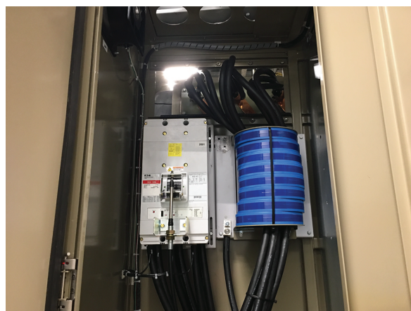
Figure 49. Adjustable circuit breaker
