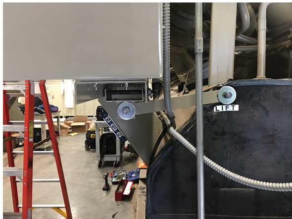
Figure 44. Fixing linkage under the C channel
