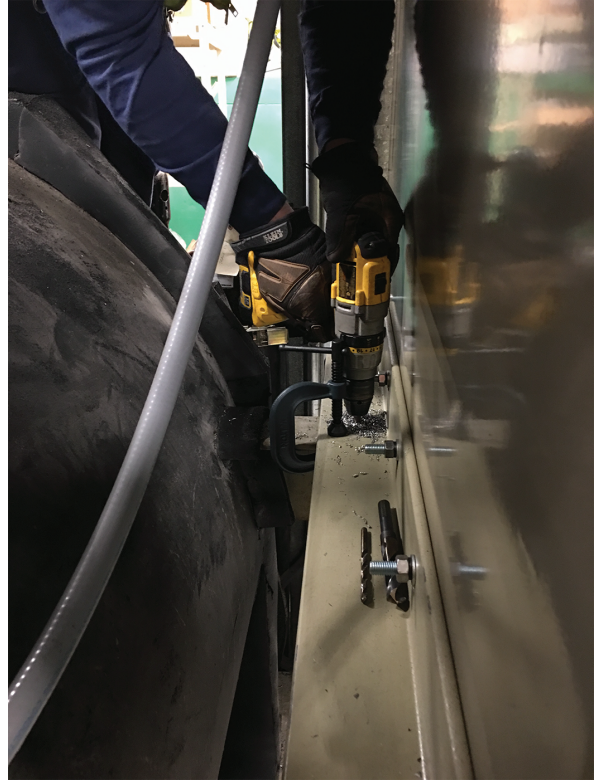
Figure 31. Installing bolts on mounting brackets on the evaporator and cabinet angle bracket
