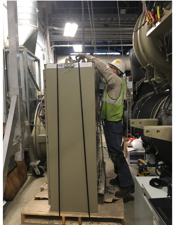
Figure 26. AFDH drive angle bracket adjustment
