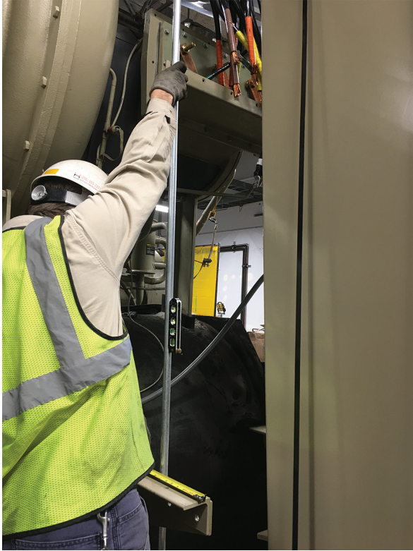
Figure 28. Starter panel brackets markings to trim extra length
