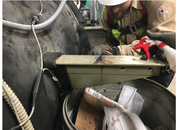
Figure 30. Starter panel brackets after trimming
