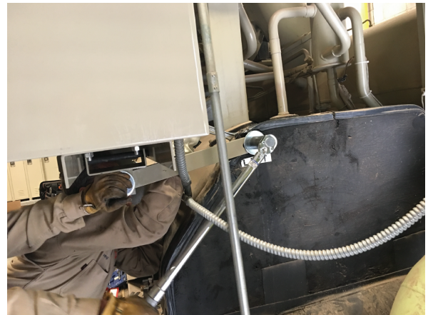
Figure 42. Install linkage subassembly into tube sheet
