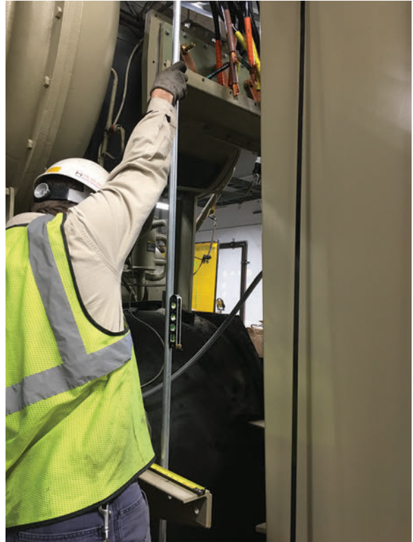
Figure 26. Starter panel brackets markings to trim extra length
