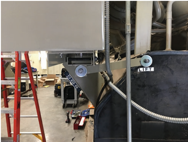
Figure 34. LiquiFlo 1.0/1.5 frame 4 mounting installation
