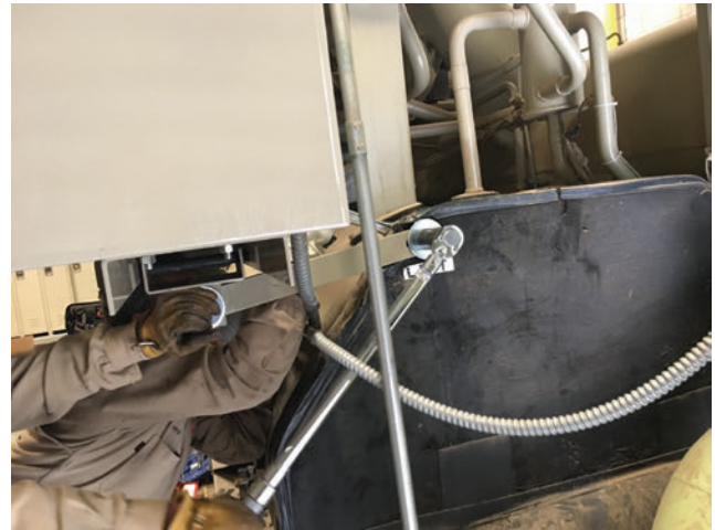
Figure 32. Install linkage subassembly into tube sheet
