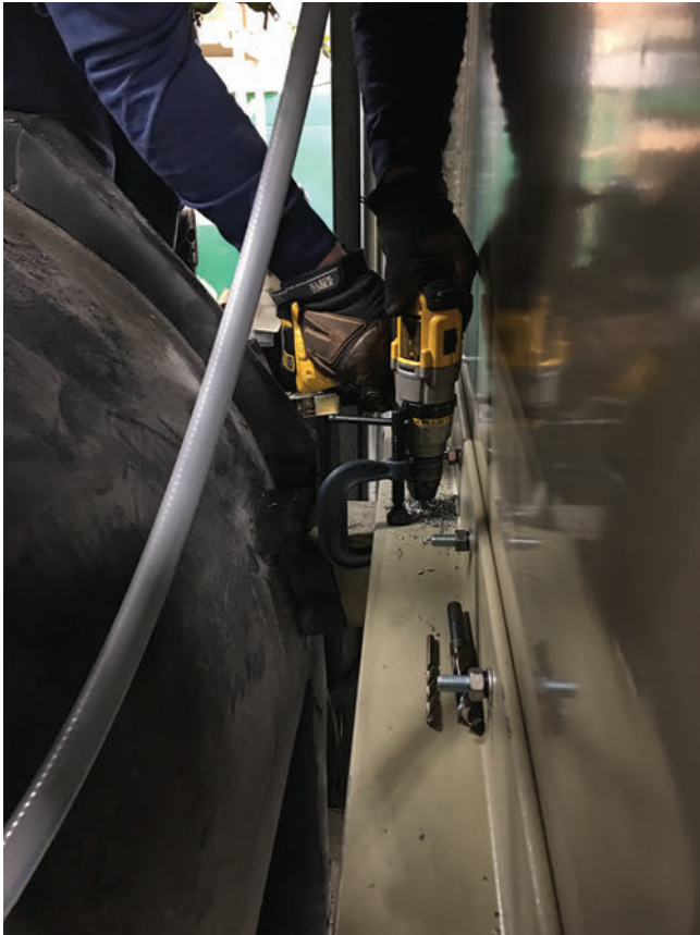
Figure 29. Installing bolts on mounting brackets on the evaporator and cabinet angle bracket
