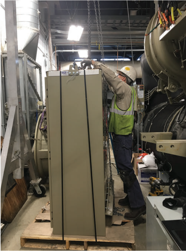
Figure 24. AFDH drive angle bracket adjustment
