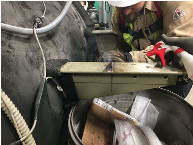
Figure 28. Starter panel brackets after trimming
