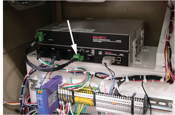
Figure 2. Electrical connections and cables removal
