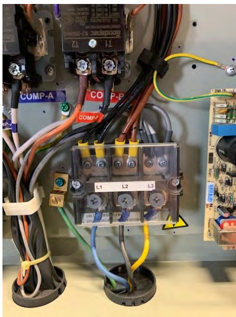
Figure 7. High voltage terminal block
