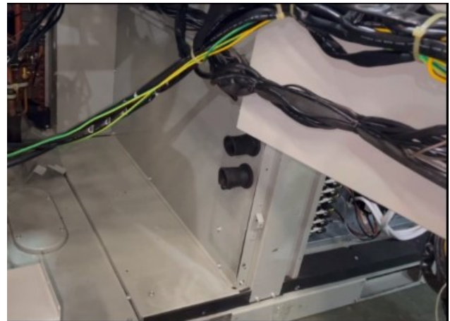
Figure 10. Rubber sheath installation
