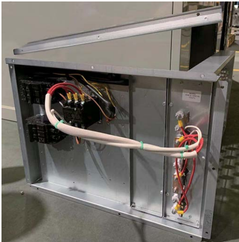
Figure 6. Remove support plate (for 7.5 ton only)
