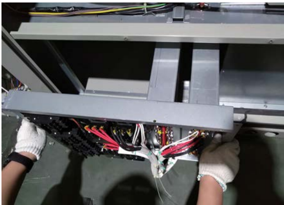
Figure 8. Electric heater aligned to screw holes
