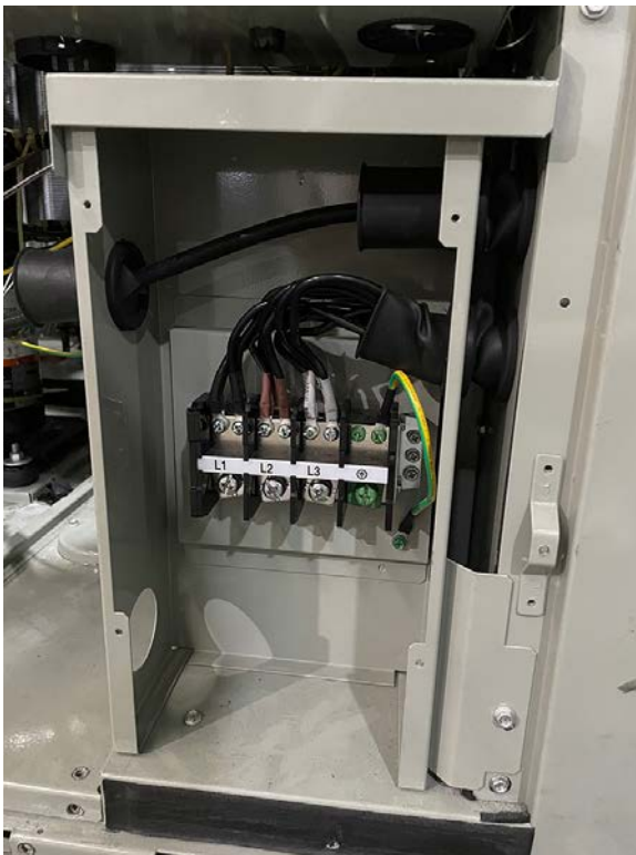
Figure 13. Connect power supply wires
