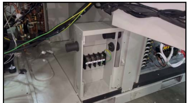
Figure 11. Control box installation
