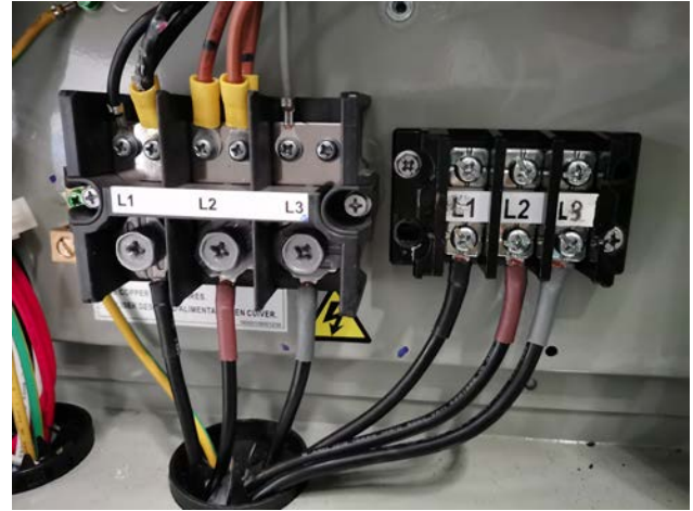
Figure 14. Power terminal block
