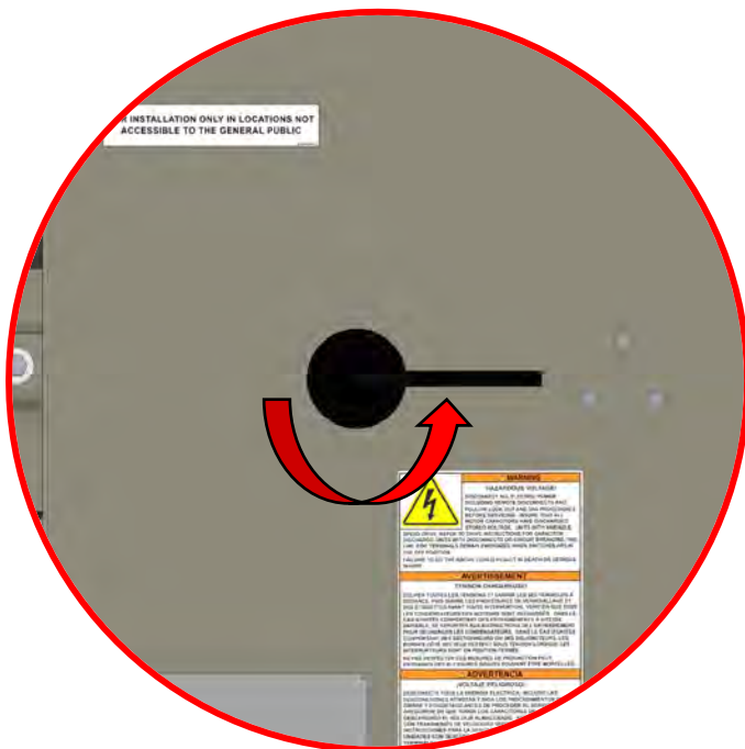
Figure 1. Turn the breaker to the Off position
