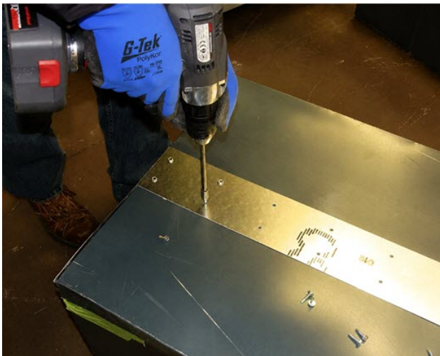
Figure 8. Fasten sheet metal over cut seam
