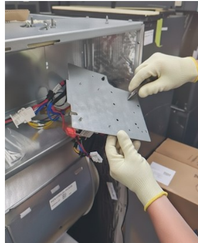
Figure 2. Mitigation control board standoff removal
