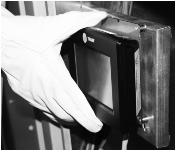
Figure 7. Mount the TD-5 human interface on the eyelet bracket (BRK04519)
