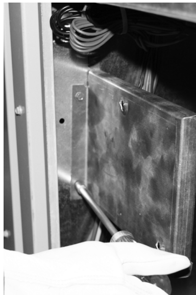
Figure 5. Installing the TD-5 human interface mounting bracket (BRK04519)
