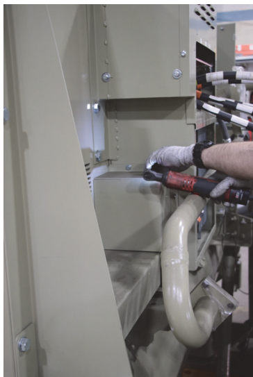
9. Remove vertical wire cover box.
