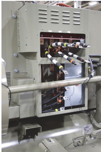
9. Remove vertical wire cover box.
