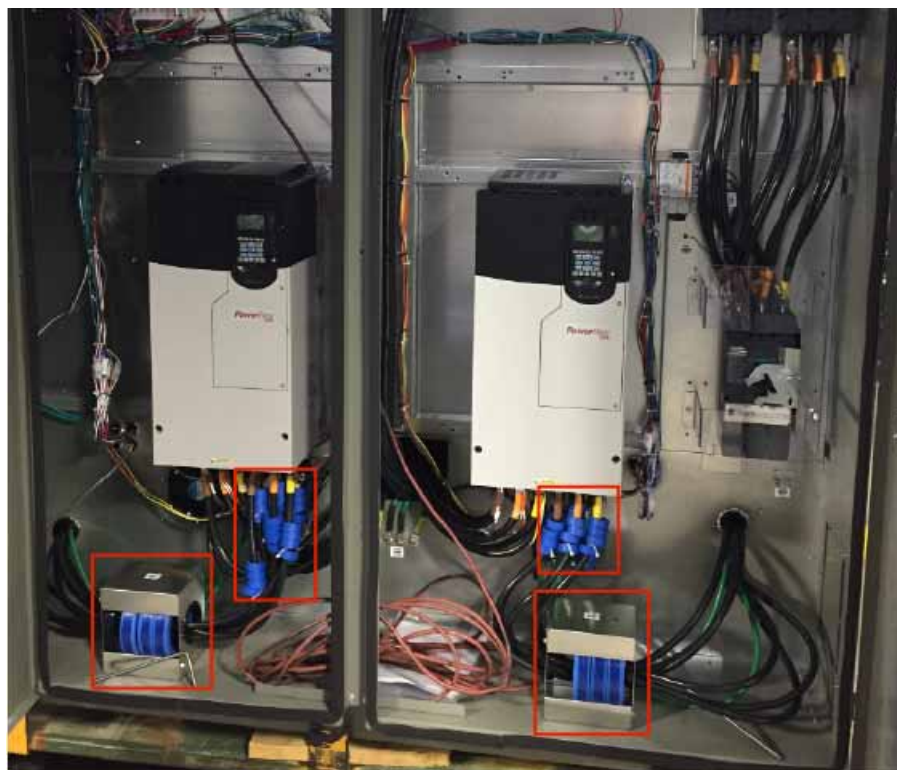
Figure 7. Output chokes locations
