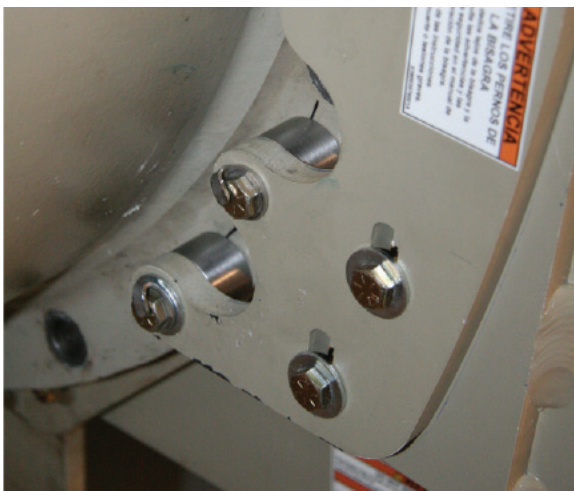
Figure 45. Fabricated waterbox cover with spacers
