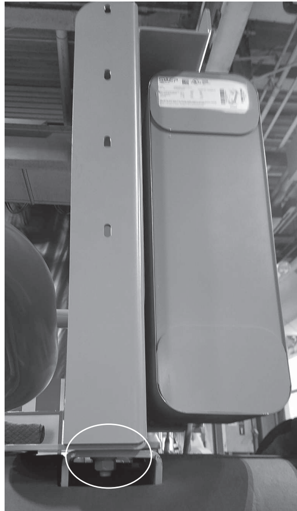
Figure 55. Unbolting the economizer 1
