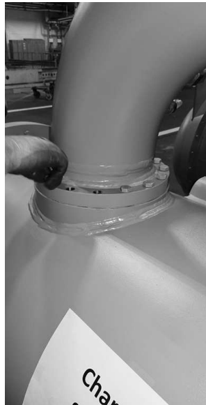
Figure 48. Removing suction elbow
