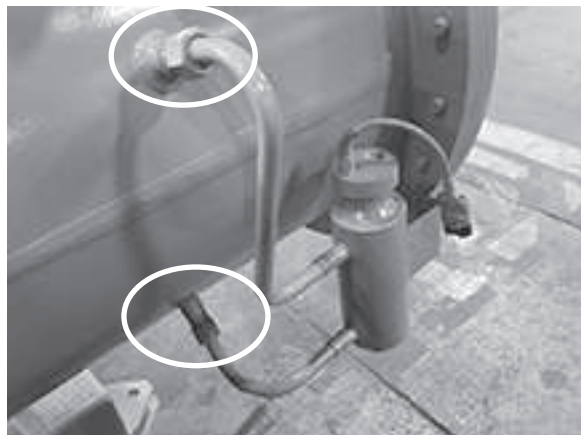
Figure 36. Removing the liquid level sensor (fittings)
