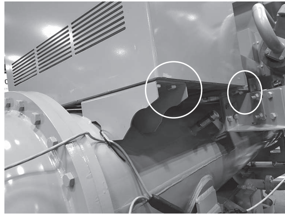
Figure 40. Removing the options panel
