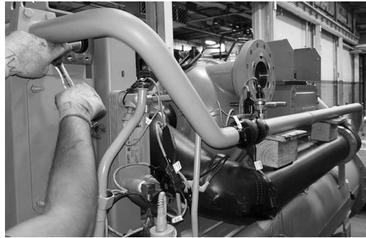
Figure 46. Securing economizer line to compressor
