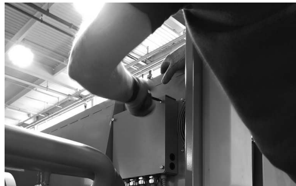
Figure 18. Disconnecting the conduits
