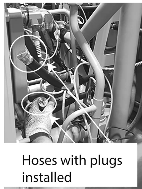
Figure 21. Plugging cooling lines
