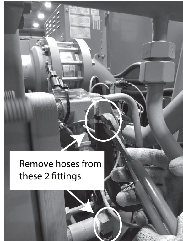
Figure 20. Disconnecting the cooling lines
