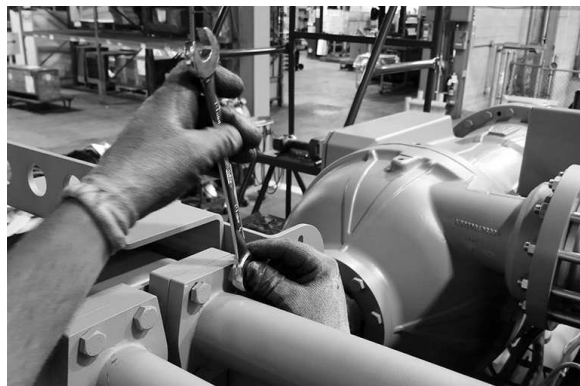
Figure 14. Disconnecting the condenser drain line from the economizer
