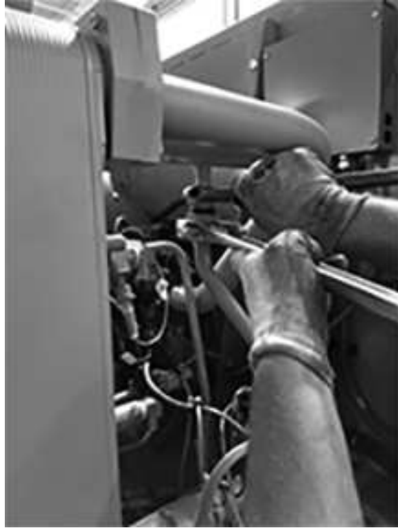
Figure 14. Disconnecting the condenser drain line from the economizer
