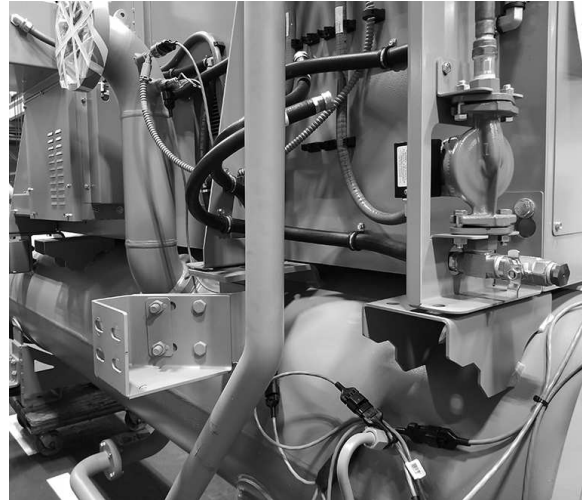
Figure 27. Removing the condenser liquid line
