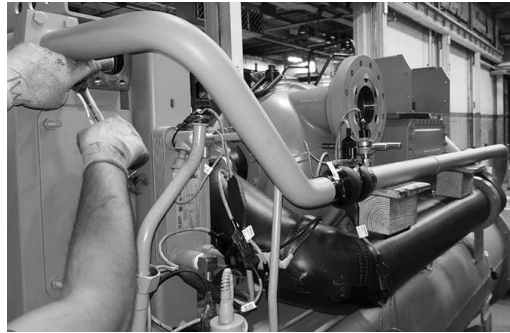
Figure 46. Securing economizer line to compressor
