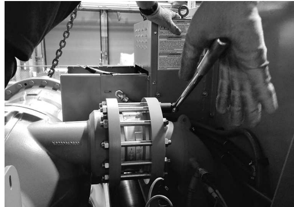
Figure 11. Check valve removal
