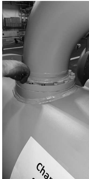
Figure 48. Removing suction elbow
