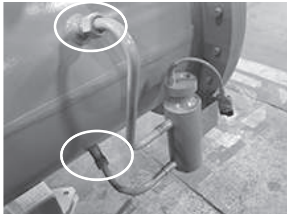
Figure 36. Removing the liquid level sensor (fittings)
