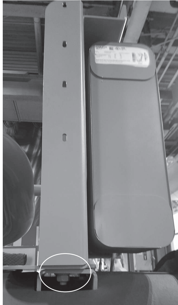
Figure 55. Unbolting the economizer 1
