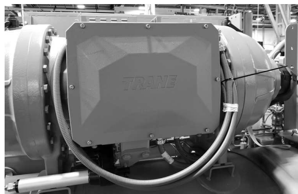
Figure 19. Securing conduits with compressor
