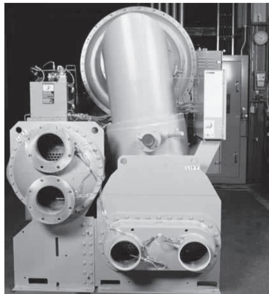
3. Remove the bolts from the flanges connecting the evaporator tube sheet and condenser shell support
