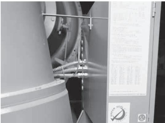
4. Two people will be needed to lift the panel clear of the chiller. Refer to [Table 11](#), p. 20 for control panel weight. Steady the panel as the top retaining bolts are removed. Then lift the panel clear. Store the panel in a clean dry area.
