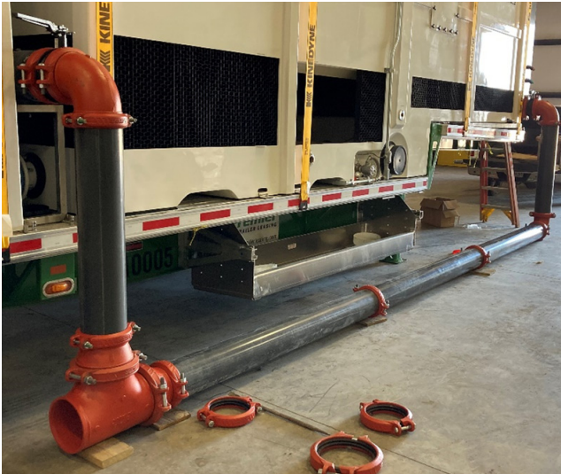
Figure 12. 1000-ton tower - assembled supply side drop piping
