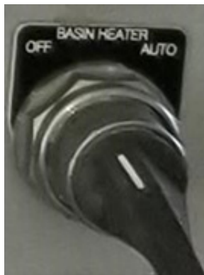
Figure 14. 270-ton cooling tower basin heater switch
