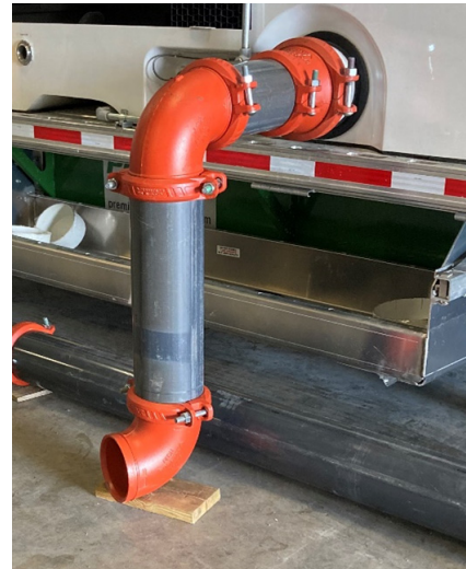
Figure 13. 1000-ton on tower - assembled suction side drop down
