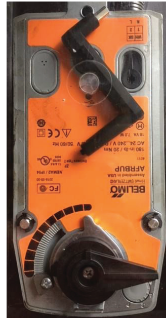
Figure 2. Spring closed position (bypass cycle)
