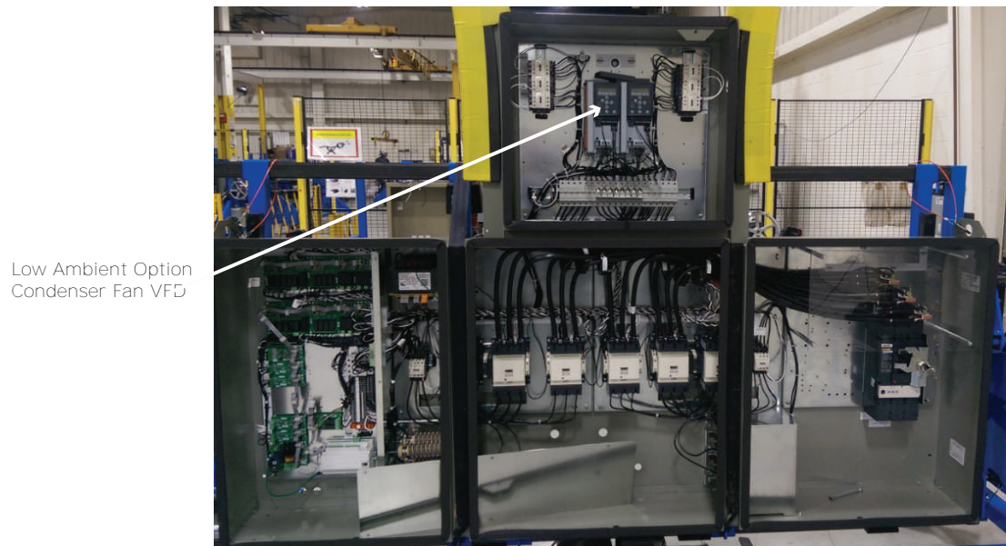
Figure 2. Typical RTAC 200 ton panel illustration and low ambient option VFD location
