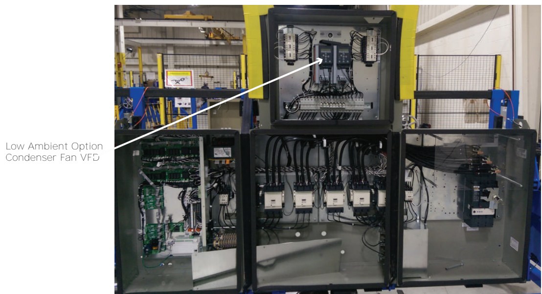
Figure 6. Typical RTAC 200 ton panel illustration and low ambient option VFD location
