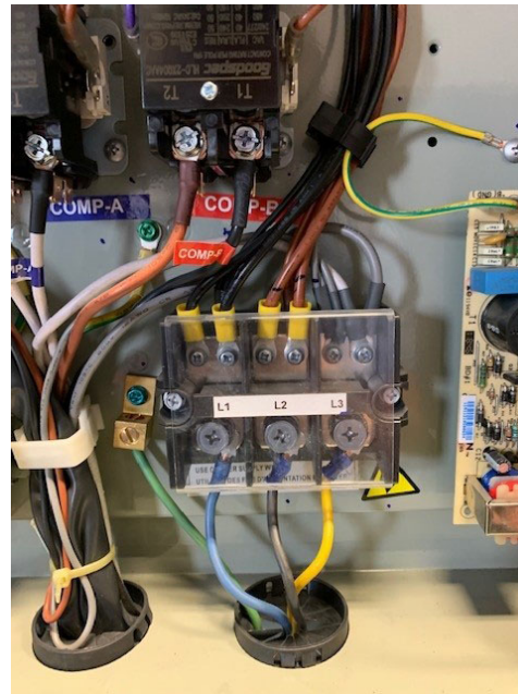
Figure 19. High voltage terminal block
