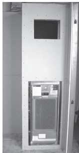
Figure 15. Install chassis centered
