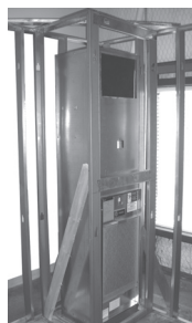
Figure 8. Mock-up of stud placement
