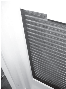
Figure 11. Air panel gasket
