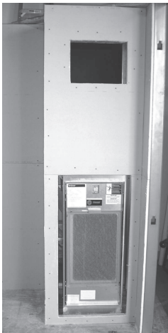
Figure 15. Install chassis centered
