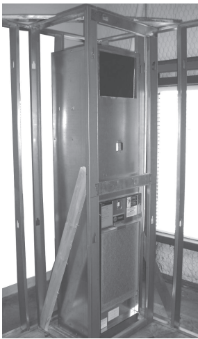
Figure 8. Mock-up of stud placement
