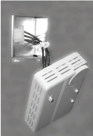
Figure 17. Zone sensor connection
