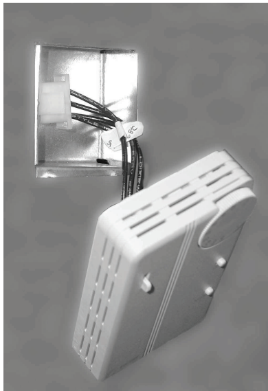
Figure 17. Zone sensor connection
