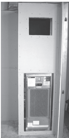
Figure 15. Install chassis centered
