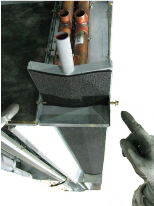
Figure 62. Removal of screws holding drain pan in place
