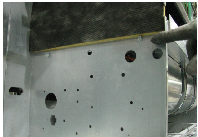
Figure 62. Loosen the two bolts (four total) at either end of the fanboard
