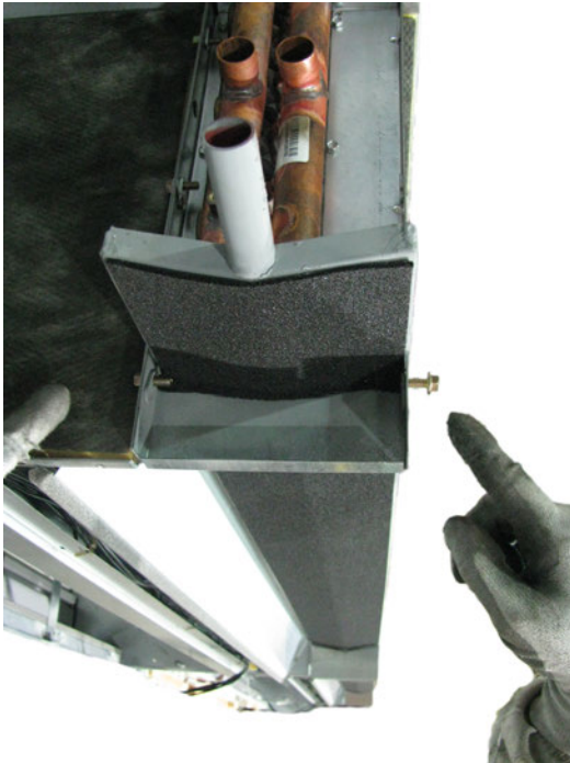
Figure 60. Removal of screws holding drain pan in place
