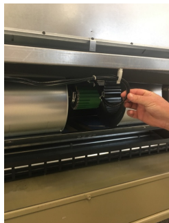
Figure 75. Disconnect fan board ground wire
