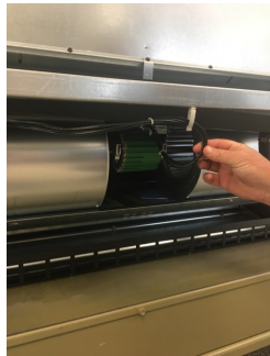
Figure 73. Disconnect fan board ground wire
