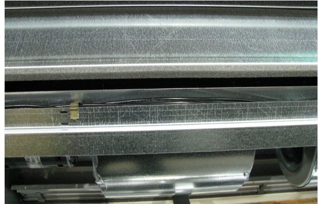
Figure 54. Tie wires from the cable chase out of the way
