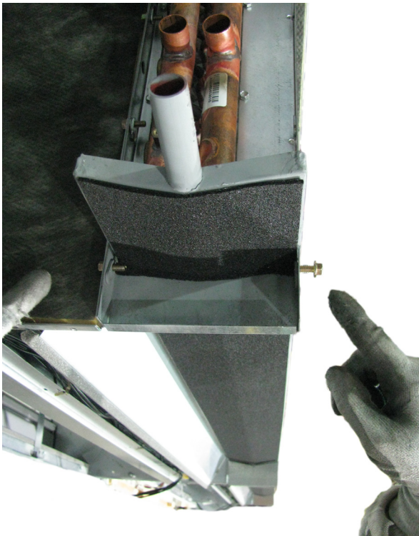
Figure 53. Removal of screws holding drain pan in place.
