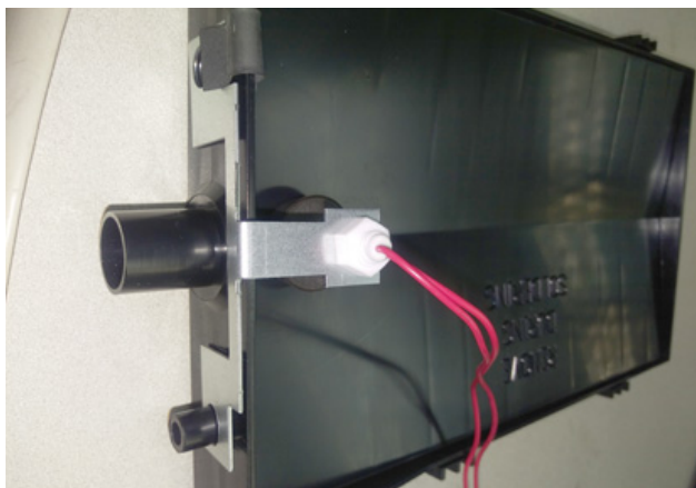
Figure 27. Condensate float switch installed in horizontal auxiliary drain pan
