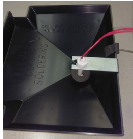
Figure 28. Condensate float switch installed in vertical auxiliary drain pan
