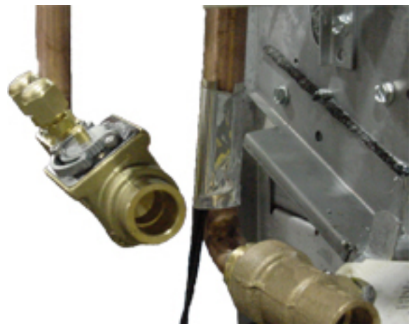
Figure 29. Attach the entering water temperature sensor to the entering water pipe as shown for changeover to work properly
