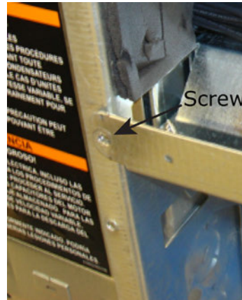
Figure 97. Fan board attachment screw
