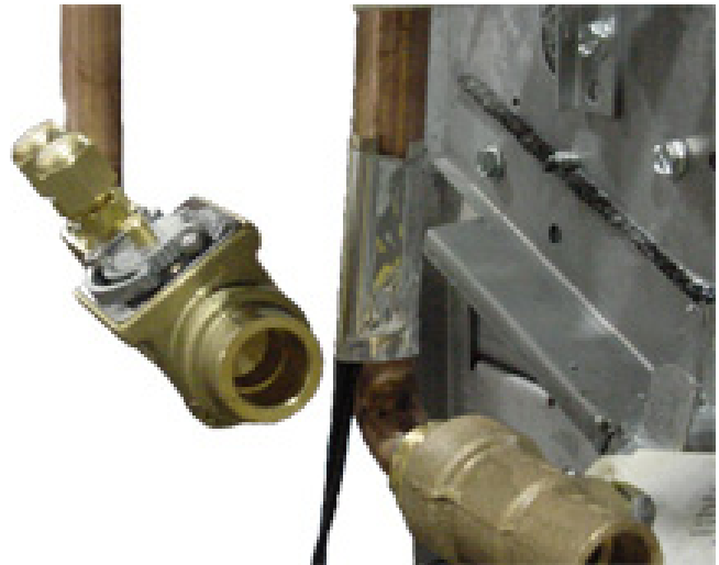
Figure 30. Attach the entering water temperature sensor to the entering water pipe as shown for changeover to work properly
