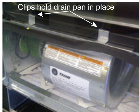
Figure 93. Clips hold drain pan to the fan board
