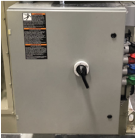
Figure 4. Externally mounted circuit breaker
