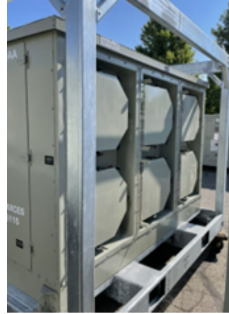
Figure 9. Return air flex duct connections
