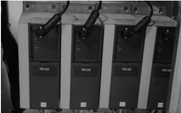
Figure 10. Trane TR150 VFDs
