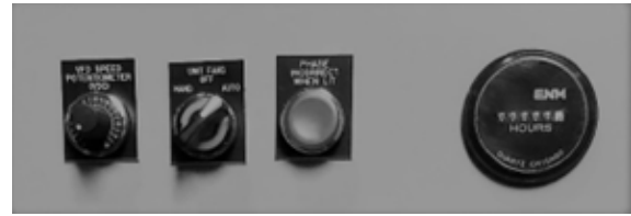
Figure 11. Speed adjustment potentiometer
