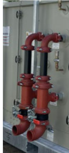
Figure 42. RSCC0030F0 - Manifold coil connections
