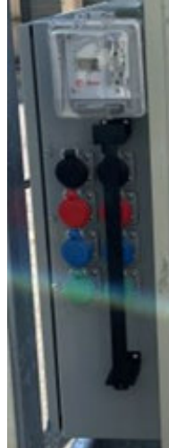
Figure 35. Input/Output cam type receptacles
