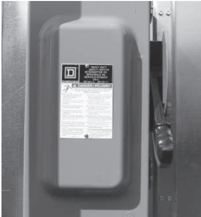
Figure 30. Internal circuit breaker
