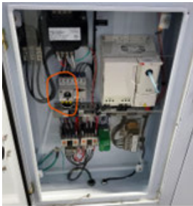
Figure 26. Internally mounted circuit breaker
