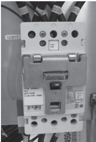
Figure 31. Externally mounted disconnect with circuit breaker
