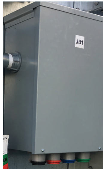
Figure 33. Series 16 cam type electrical connections
