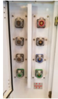
Figure 28. Input/Output cam type receptacles
