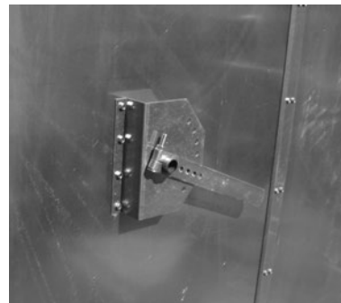
Figure 45. Handle to control linked dampers
