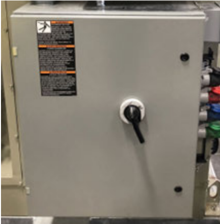
Figure 34. Externally mounted circuit breaker
