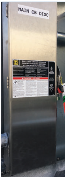
Figure 31. Externally mounted disconnect with circuit breaker
