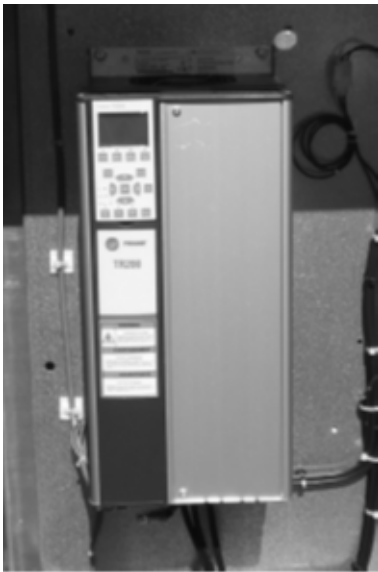
Figure 48. Trane TR200 VFD
