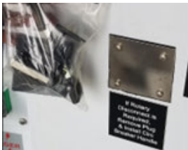
Figure 27. Removable disconnect handle
