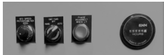
Figure 51. Speed adjustment potentiometer
