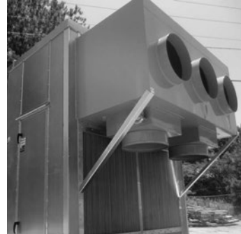
Figure 45. Handle to control linked dampers
