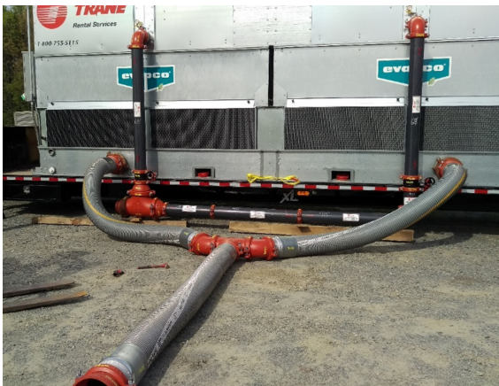
Figure 10. Cooling tower - assembled piping kit
