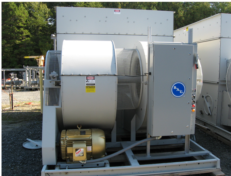
Figure 5. CT motor control panel end
