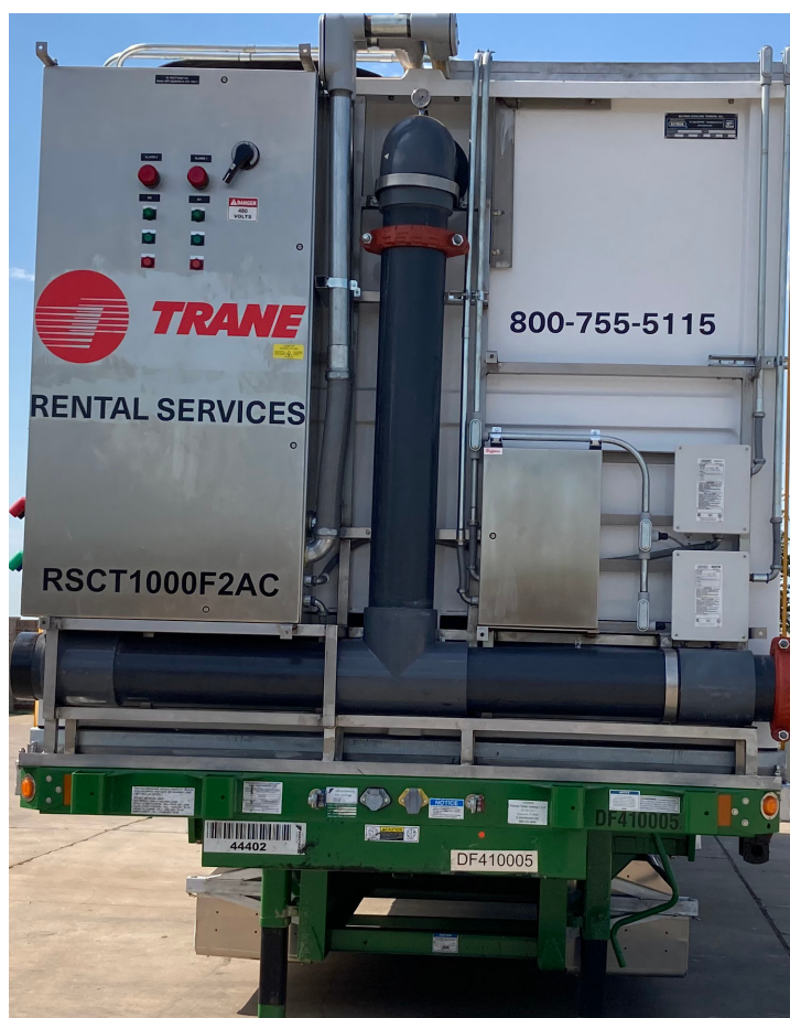
Figure 7. 1000-ton CT control panel end
