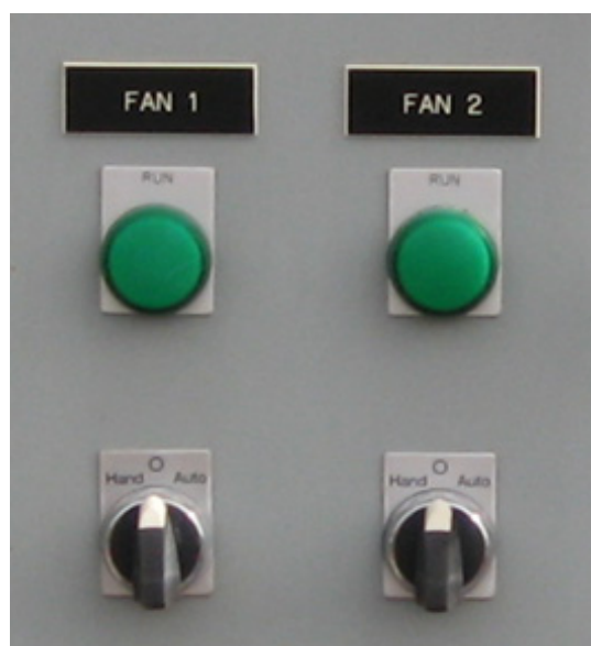
Figure 18. Cooling tower fan switch
