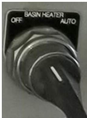
Figure 14. Cooling tower basin heater switch
