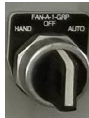
Figure 15. Cooling tower fan switch
