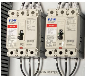
Figure 21. Cooling tower basin heater breakers
