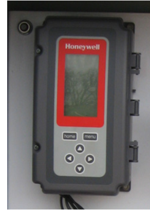
Figure 19. Cooling tower temperature control
