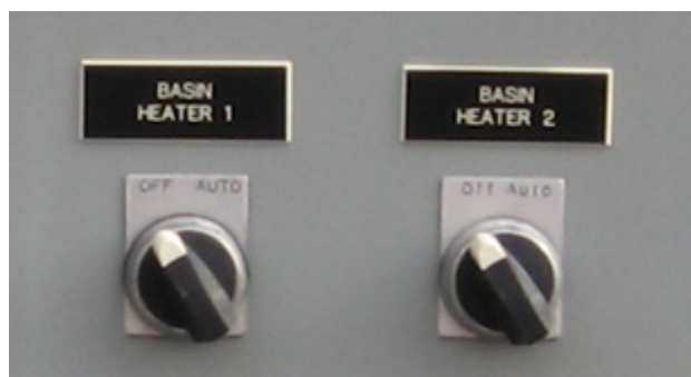
Figure 17. Cooling tower basin heater switches
