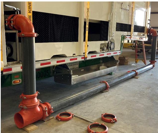
Figure 12. Assembled supply side drop piping
