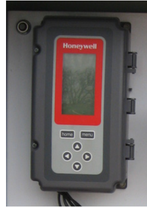
Figure 19. Cooling tower temperature control
