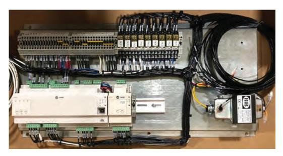
4. Install the new back plate to the main electrical panel with provided sheet metal screws.
