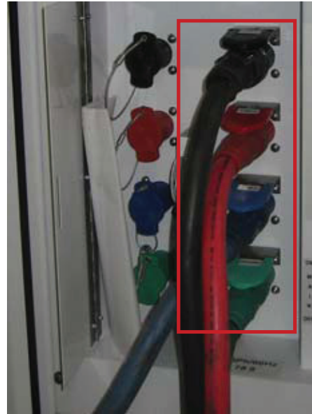
Figure 6. Cam-type electrical connections - pin connectors
