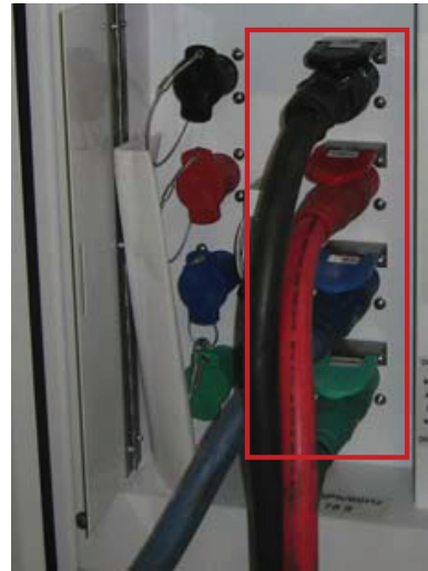
Figure 21. Color coded (black, red, blue, and green) cam-type electrical connections
