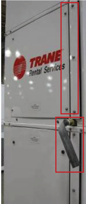
Figure 19. Tent clamps and condensate kazoo tube drain
