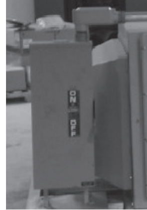
Figure 2. Main unit disconnect
