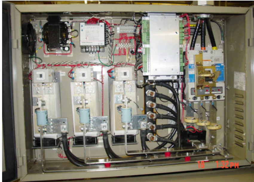
Figure 12. Photograph of A515 solid state starter
