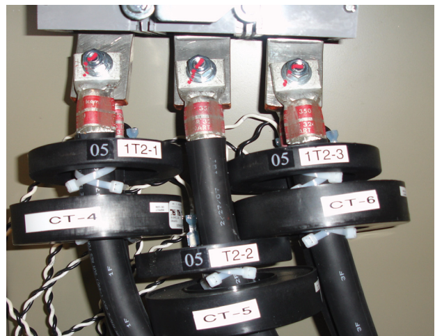
Figure 39. RTHD - Installation of CTs
