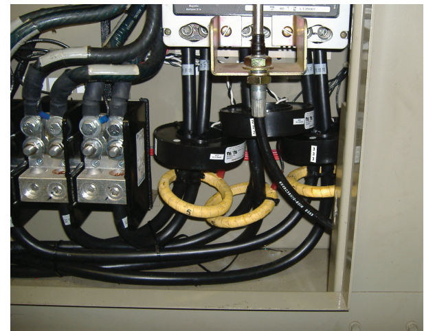
Figure 39. RTHD - Installation of CTs
