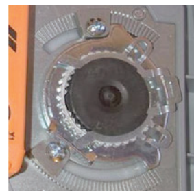
Figure 54. By-pass valve setting photo
