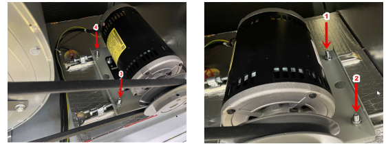
Figure 25. Tighten plate bolts
