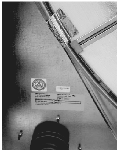
Figure 104. Link belt installation
